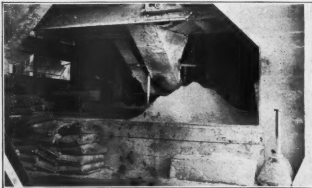
Mixing Machine in Brick Plant
